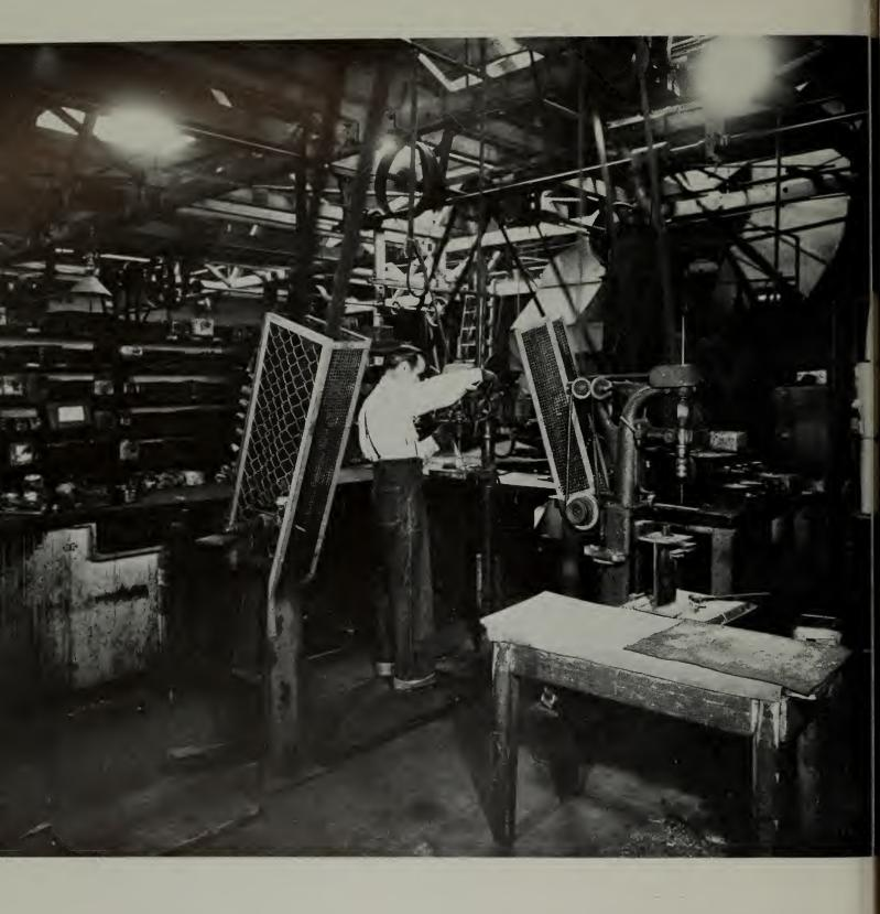
The operator cleans out the oil holes by use of a drill press as shown in this picture.
